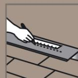
Once again, make sure that there is an 8 to 10 mm expansion joint. Take the joint into account when measuring and sawing the planks of the final row lengthwise.
