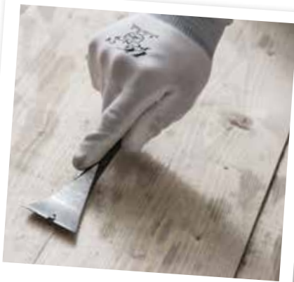
REMOVE LOOSE NAILS
